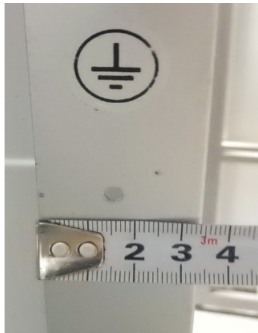
Detail view of grounding hole
